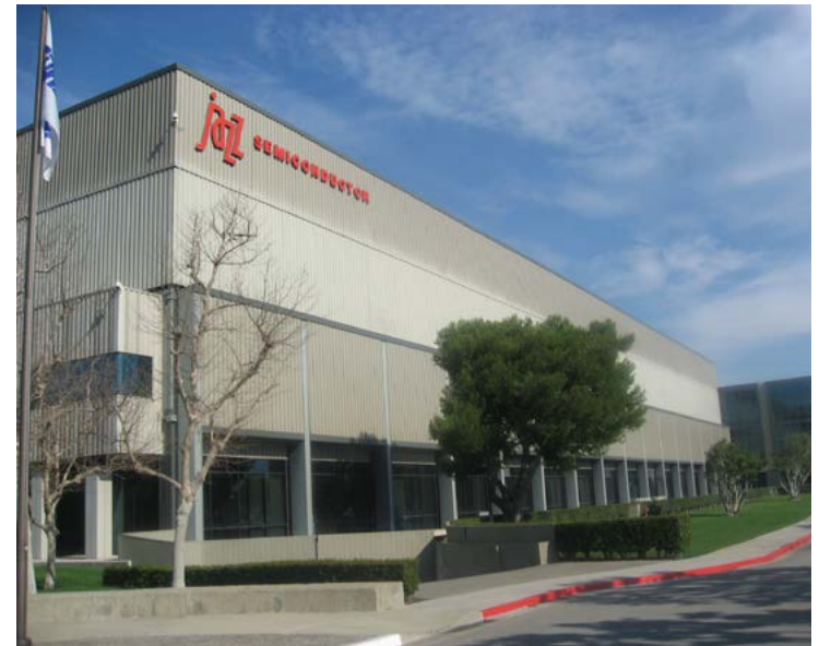
Figure 3-10: Existing TowerJazz Building
