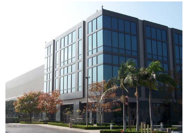
Figure 5-1: Existing TowerJazz Building
