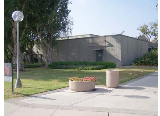
Figure 2-1: Half Dome building
